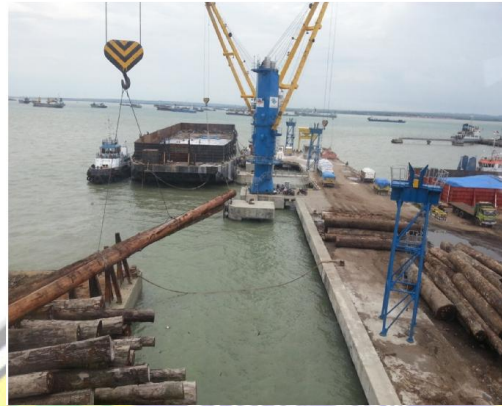
Gambar 2.1 Level Luffing Gantry Crane (LLGC).
