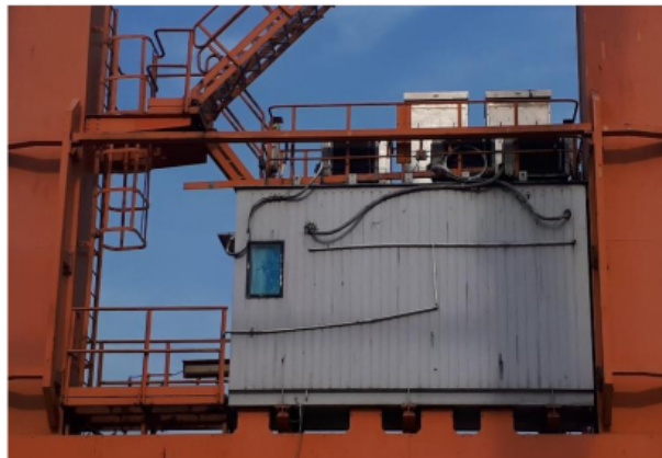
Gambar 2. 3 Bagian Electric Room
